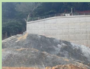
斜坡淋漿 Shotcrete in Slope
