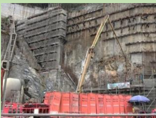
設置隔音屏障 Installation of Noise Barriers
