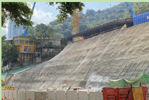
斜坡鞏固工程 Slope Stabilizing Works
