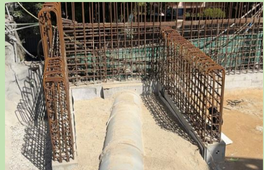
渠務工程 Drainage Construction Works
